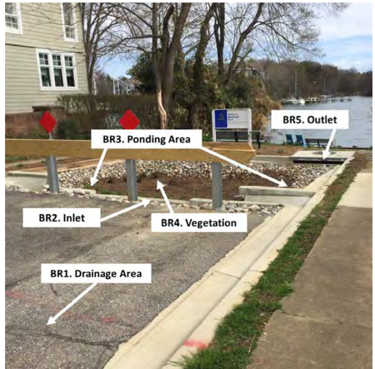
Figure 2.7.1. Key Areas for Level 1 Inspection of Bioretention
